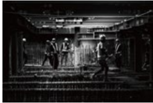
Dimension Space/Chan-Nok-Hang - Workers Under Secure Support
