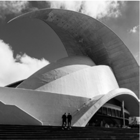
Carmen R Perez - Tenerife Auditorium Silver in Architecture, Buildings
