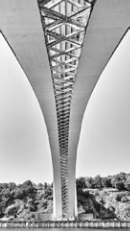
Glenn Goldman - Arrabida Bridge Silver in Architecture, Bridges
